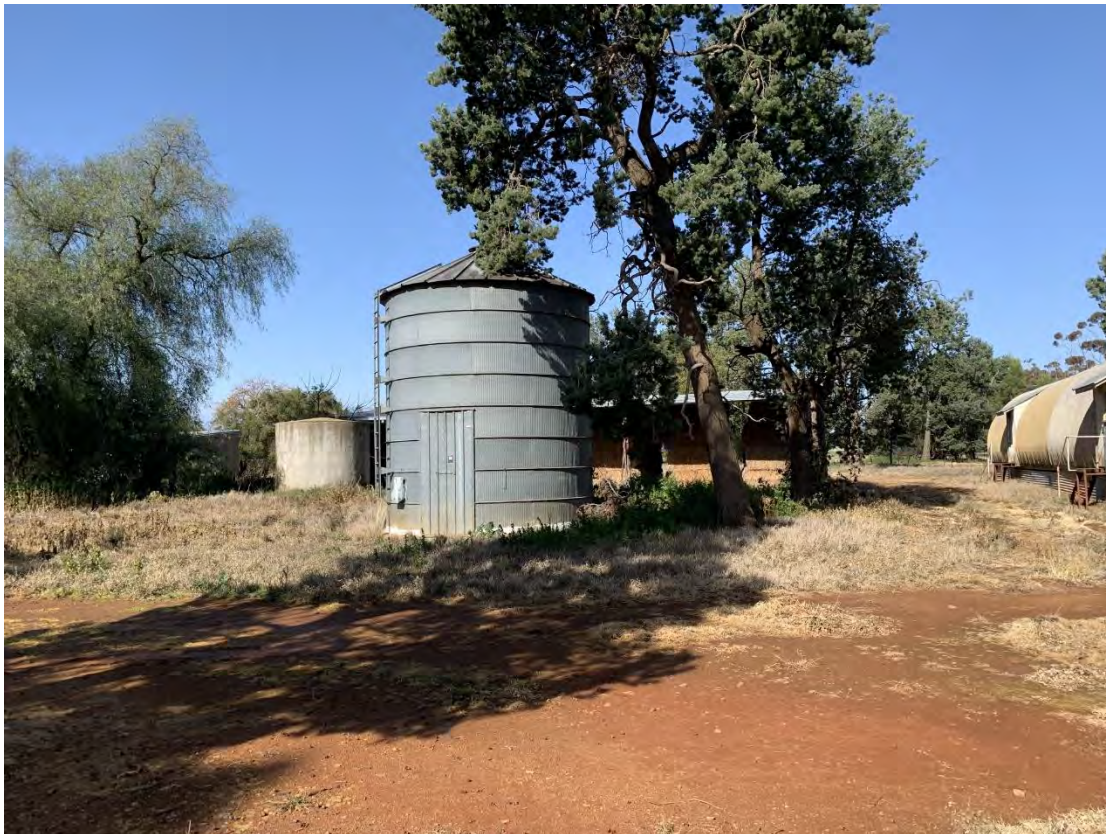
Photograph 14: The slab on grade steel silo.
